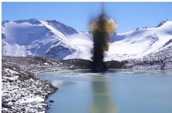
Works on the expansion and deepening of evacuation channels on moraine lakes are carried out using drilling and blasting.
