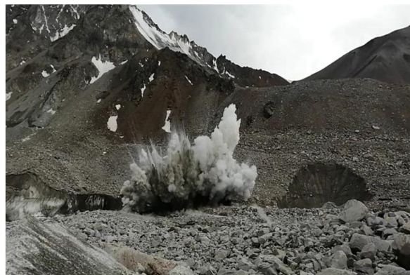
Works on the expansion and deepening of evacuation channels on moraine lakes are carried out using drilling and blasting.
