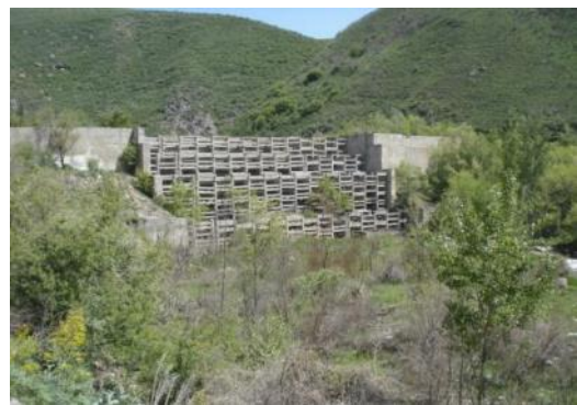
stopping reinforced concrete grid dam on the Kaskelen river (A. P. Medeu et al., 2020)
