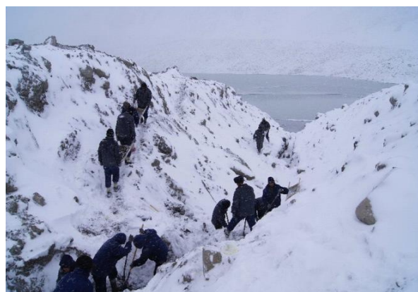
Works on the expansion and deepening of evacuation channels on moraine lakes are carried out using drilling and blasting.
