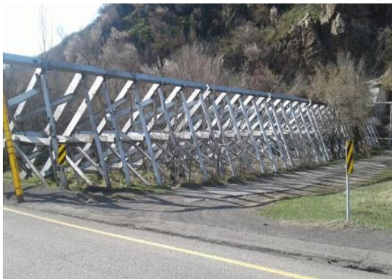
Mudflow catcher struction on the Kishi Almaty River
