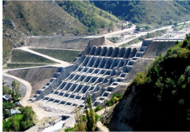
Mudflow retention dam on the Talgar River
