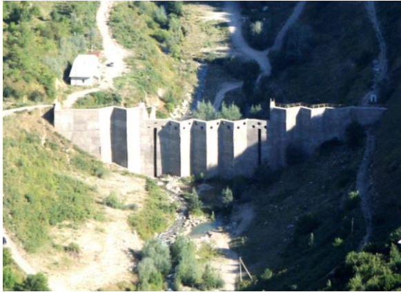
Anti-mudflow dam on the Kargaly River
