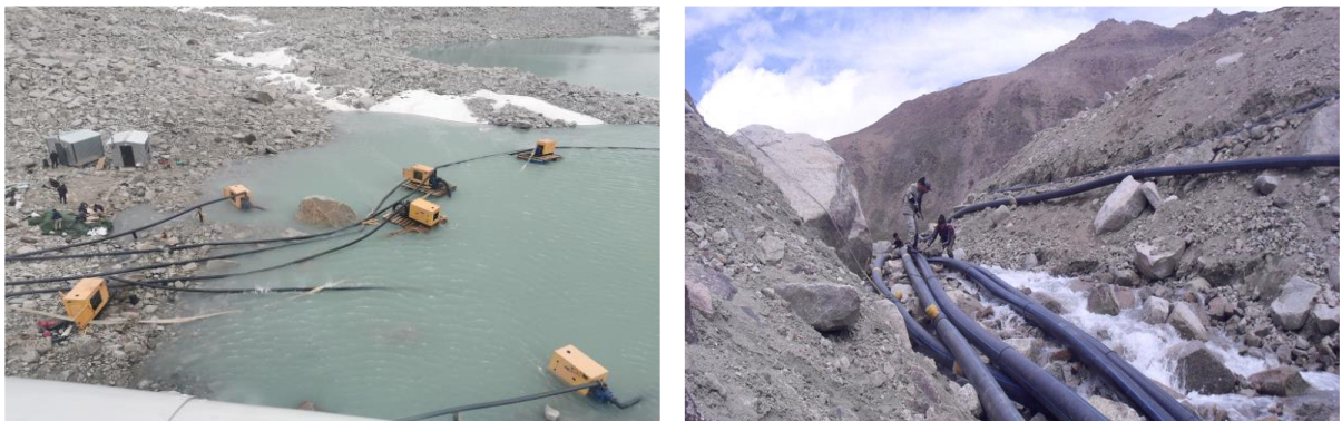
Lake emptying using a water pump
