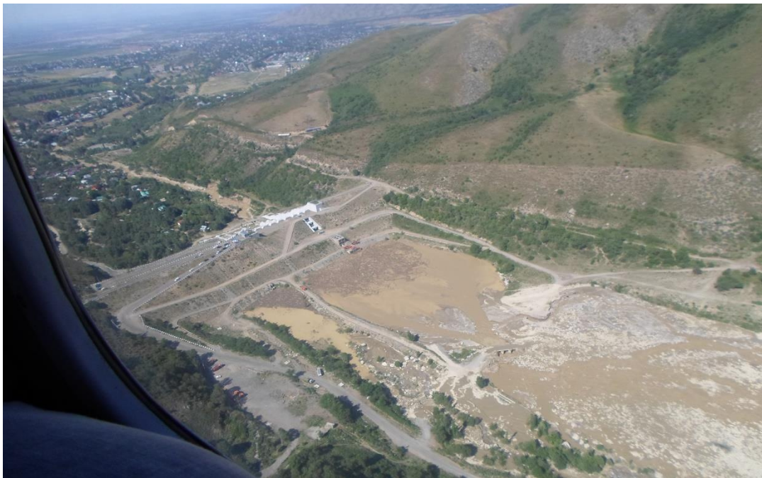
Figure 6. Partially Filled Sediment Storage Basin Before the Talgar Dam.
