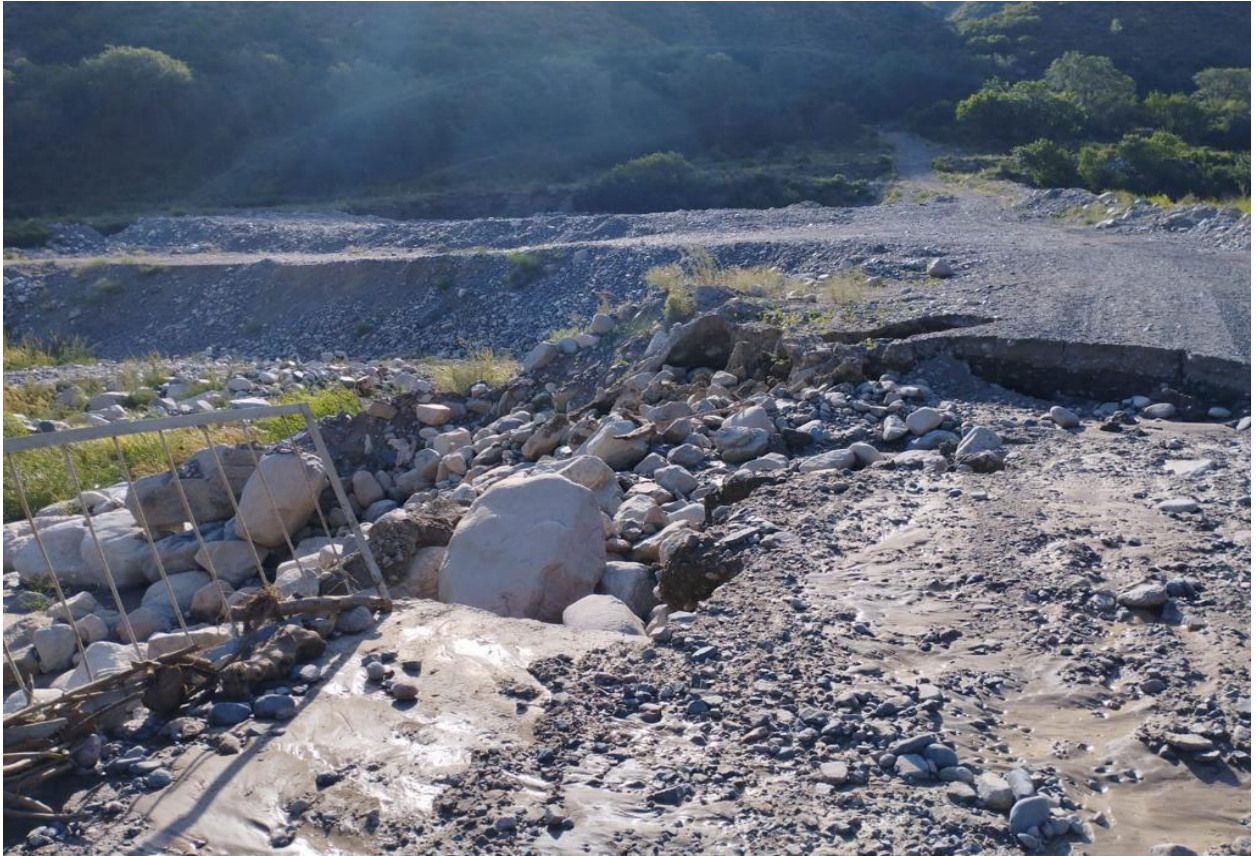
Figure 4. Consequence of mudflow on 21 July 2023 at the dam of Talgar river (photo 22.07.2023 by 'Kazselezaschita').
