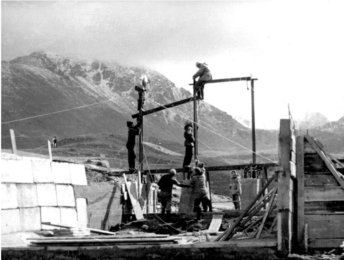
Fig. 4. Construction of the dam outlet works in the Chemolgan River basin.
