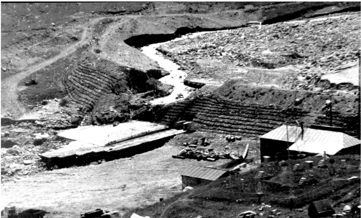
Fig. 2. Gabion dam opening after the debris flow of 15 July 1973.
