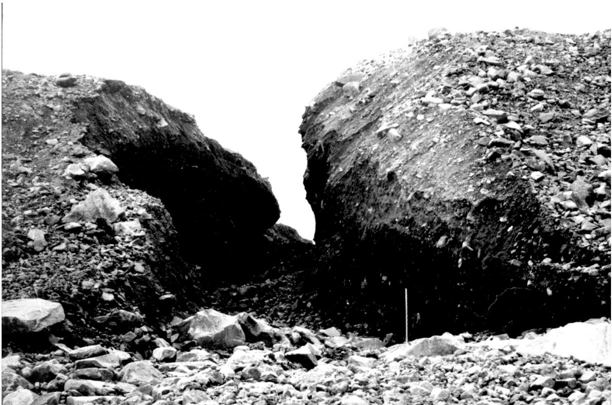
Fig. 2. Opening in the dam of lake No 13 (view from the downstream wall of the dam).
