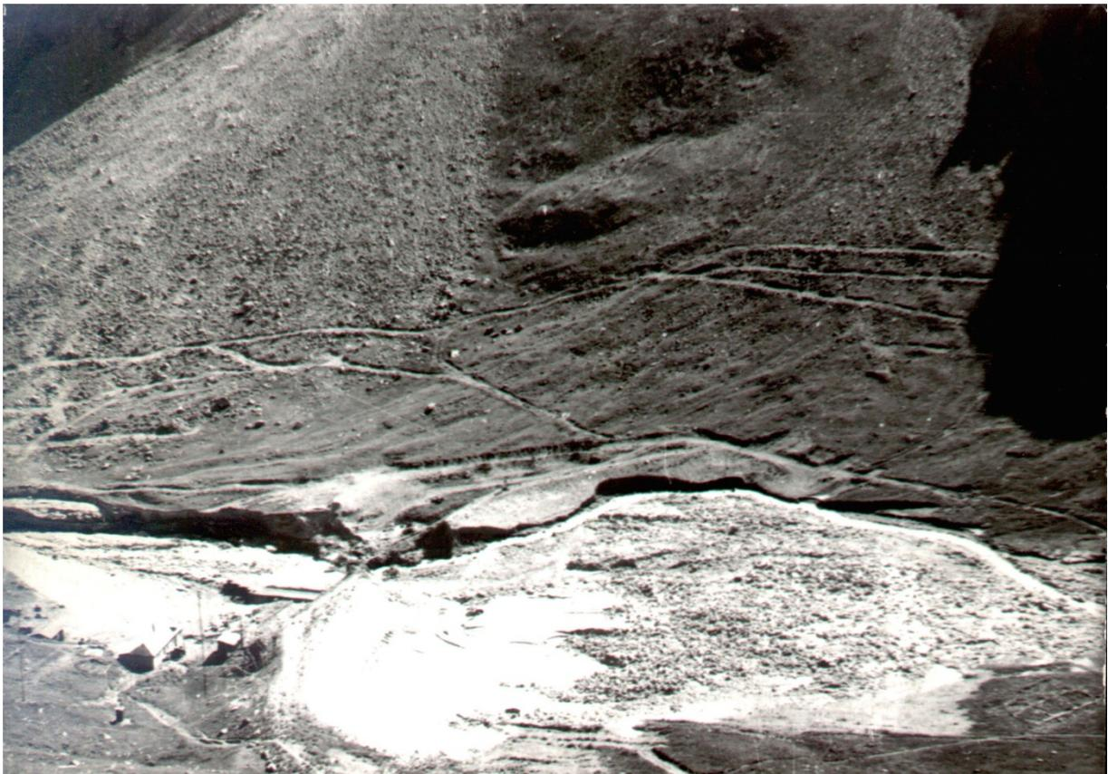
Fig. 7. The gabion dam after the outburst, view from the upper reach.
