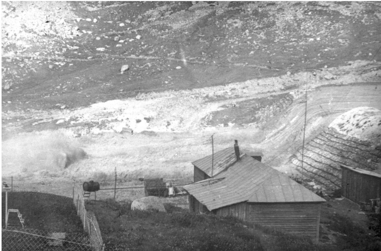
Fig. 8. Flow of the outburst flood through the crest of the gabion dam (photo by V. Ya. Bosharimov).
